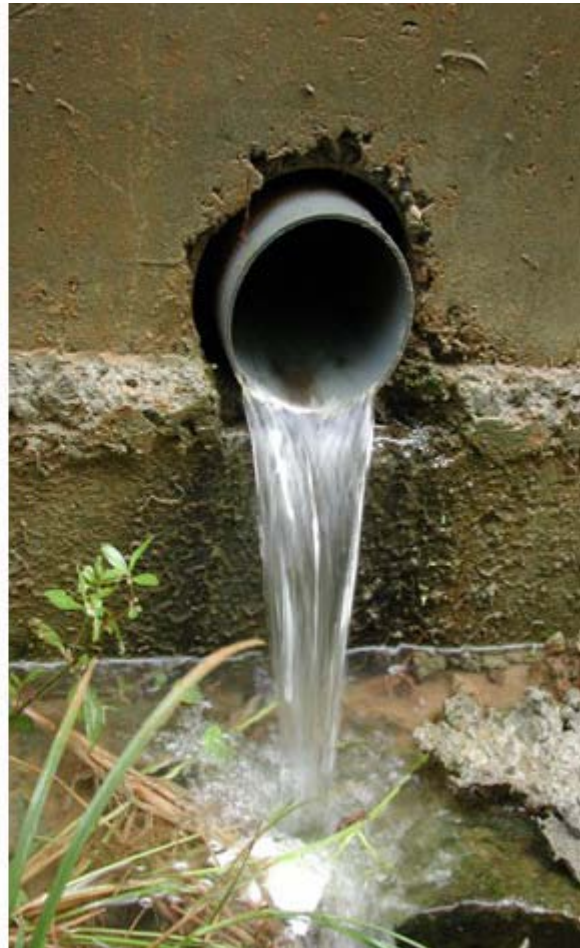
WATERBELT INSTALLED AS A BACK DRAIN FOR A RETAINING WALL IN A VERTICAL CONFIGURATION. THE COLLECTION OF WATER DURING A TYPHOON RESULTS IN A HEAVY DISCHARGE
