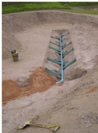
BUNKER DRAINAGE REPLACEMENT
