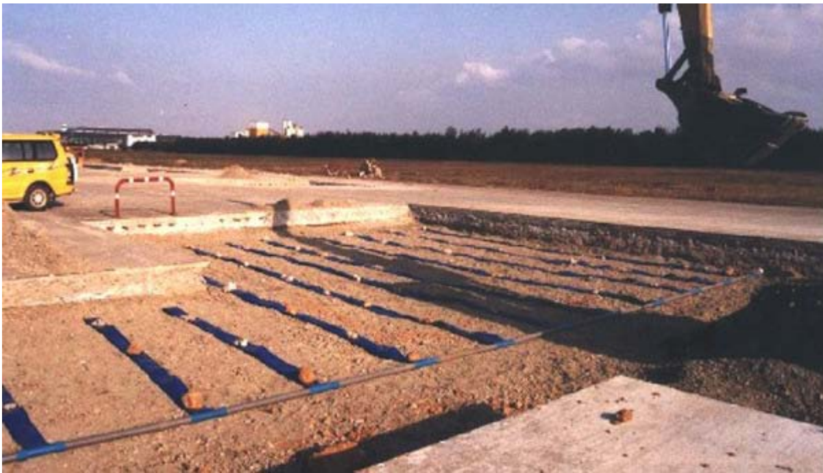
APRON SLAB DRAINAGE
