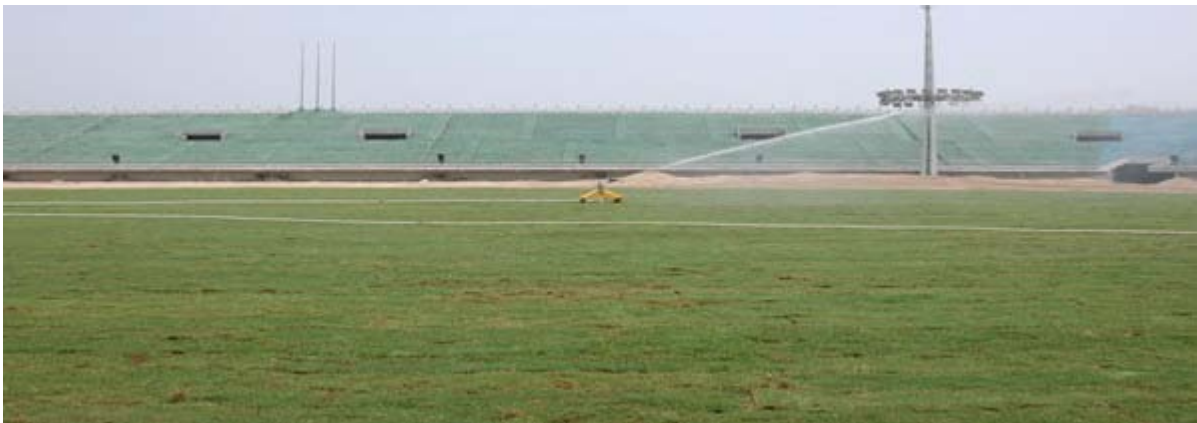
BACKFILL AND SOD
