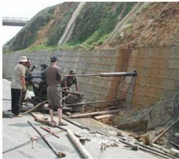
ASSEMBLED PIPES READY FOR INSTALLATION
