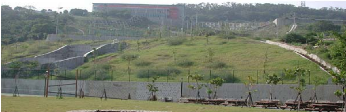
RETAINING WALL INSTALLED TO STABILIZE SLOPE
