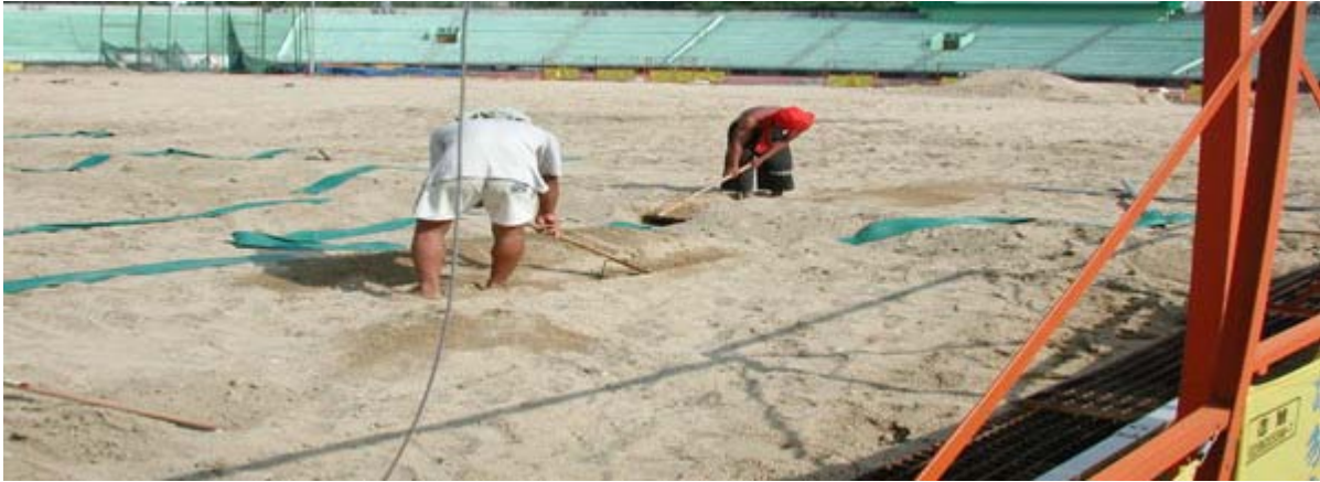
INSTALLING WATERBELT FOR SPORTS FIELD
