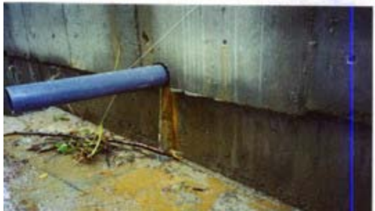
WATERBELT INSTALLED AS A BACK DRAIN FOR A RETAINING WALL IN A VERTICAL CONFIGURATION. THE COLLECTION OF WATER DURING A TYPHOON RESULTS IN A HEAVY DISCHARGE
