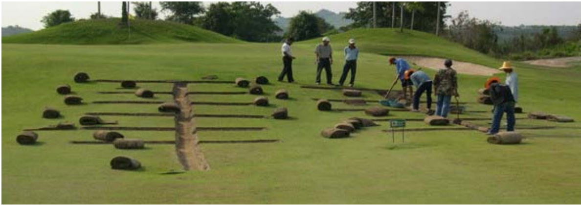
FAIRWAY DRAINAGE REPLACEMENT
