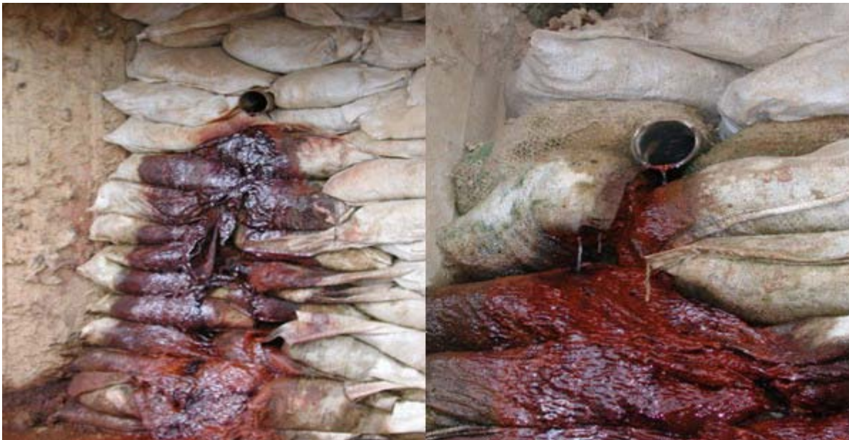
TRADITIONAL DRAINAGE BLOCKED BY LIMOLITE AFTER ONLY 15 DAYS
