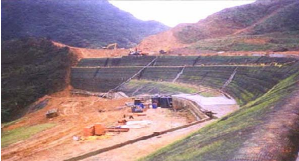
RETAINING WALL OF TAWULOOK HIGHWAY (TAIWAN)
